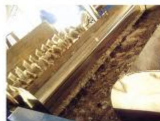
PE/PP WASHING TANK
